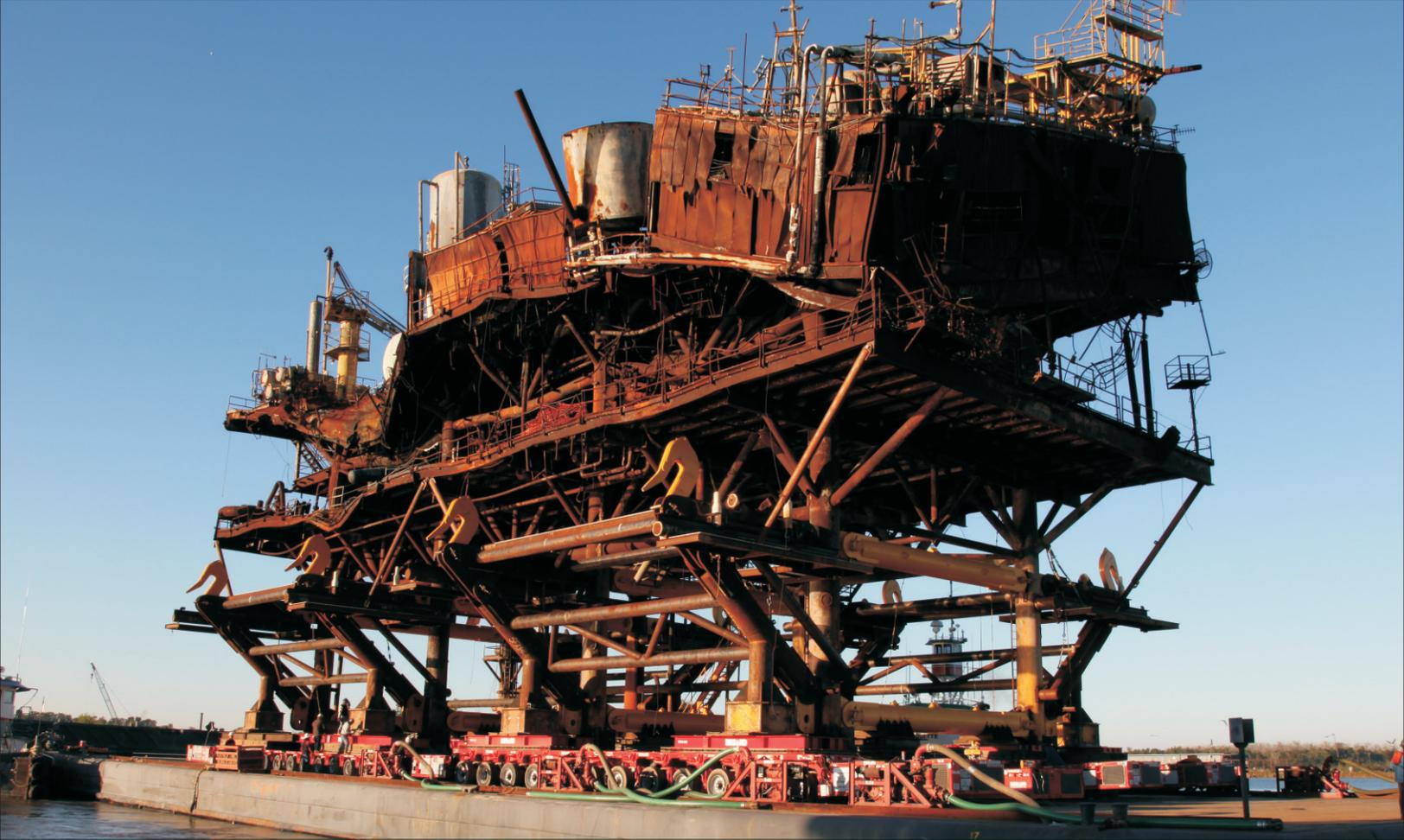
Loading and offloading offshore platforms is just about an everyday occurrence at Berard. This one however was just a little different. During one of the recent hurricanes this deck weighing 2600 tons developed a “minor” fire. Once removed from it’s foundation offshore and transported to the clients facility in Gibson Louisiana, the Berard Team took action to make this final part of the move a safe and successful one.
